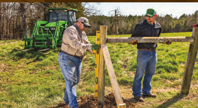
Replace A Wire Fence End Post And H-Brace
